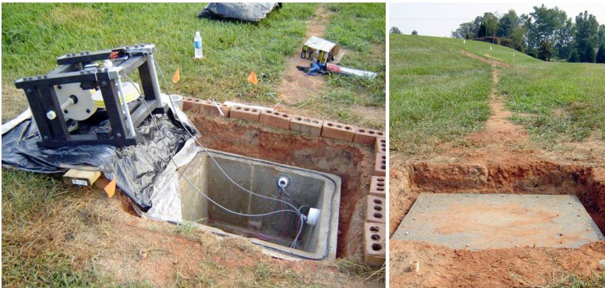
Figure 3. Installation of prototype sensor. Sensor consists of two orthogonal coils, visible as white spools mounted in the plastic framework. Second photo shows the B (middle) sensor vault. The C sensor's location is still apparent in the background as the grass has not yet covered the signal cable trench and vault.
